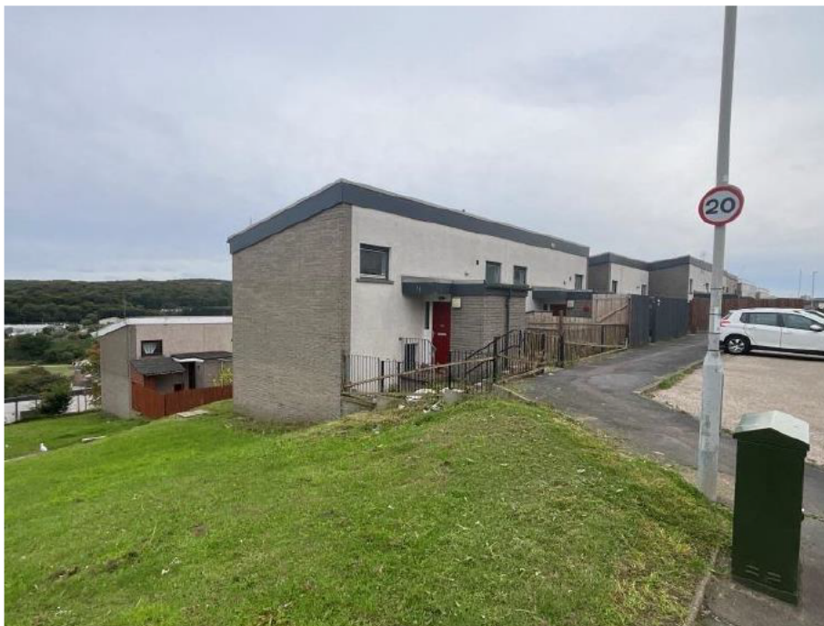
Figure 7: Refurbished 'flat' roof system
